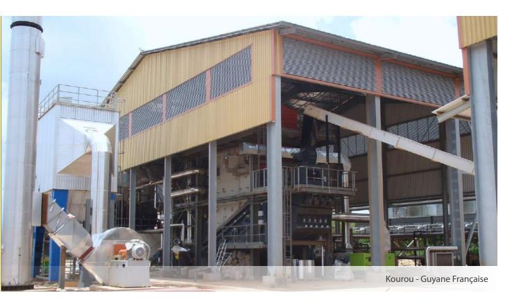
Wood consumption only covers the biomass power plant in Kourou. Wood waste is the main raw material used. It consists of off cuts, splinters or logs to be milled, wood chips and sawdust. In 2019, Voltalia recovered 29,388 tonnes of wood waste to operate its biomass power plant in French
