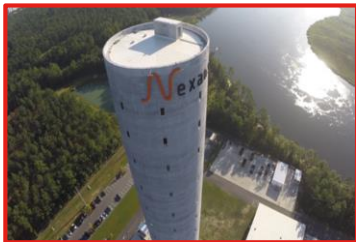
Goose Creek Plant, South Carolina, USA Land High Voltage Cables Update for Submarine High Voltage (2020)
